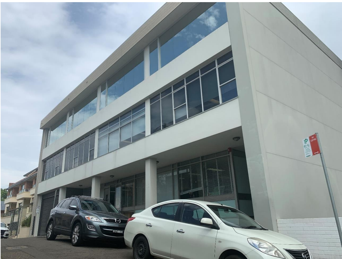
Figure 11 – 271-273 Alfred Street, rear frontage at Little Alfred Street.
