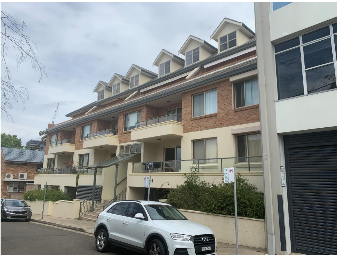
Figure 9 – 4 Little Alfred Street, principal frontage.
