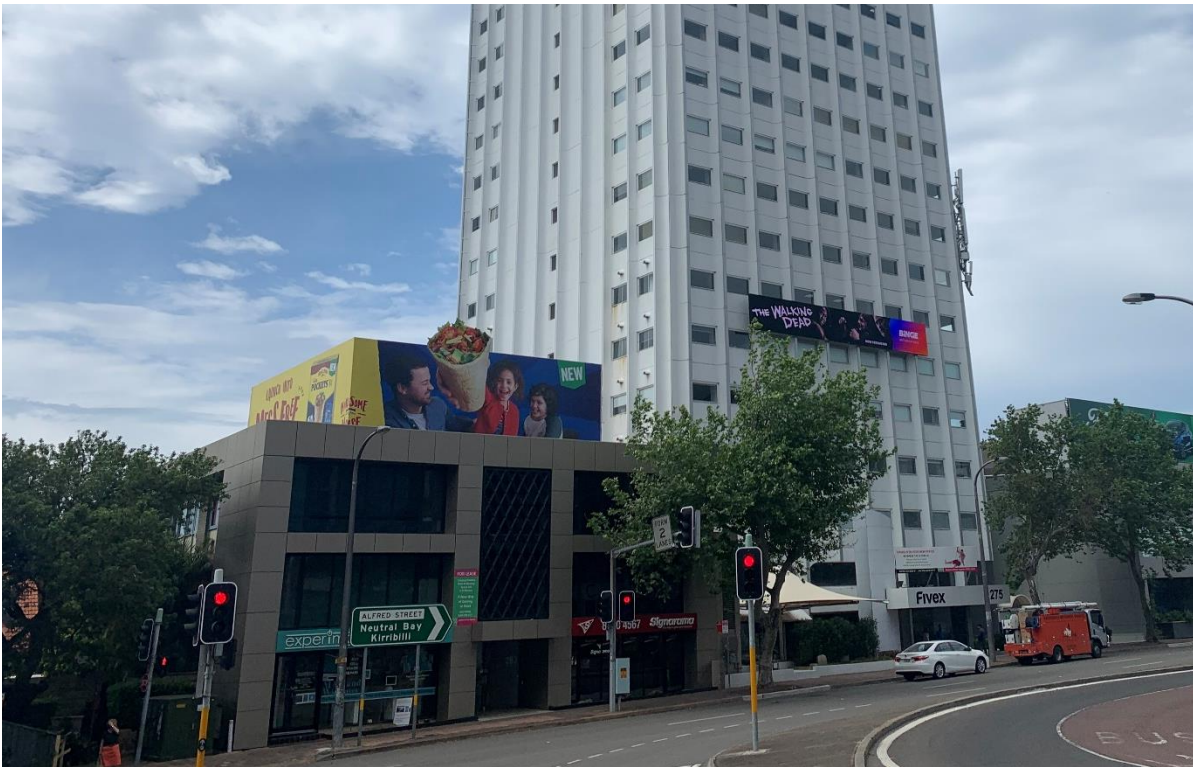
Figure 13 – 283 Alfred Street, principal frontage.
