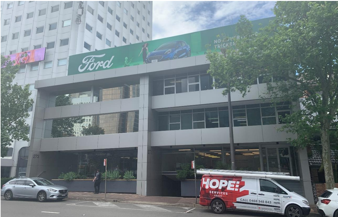
Figure 10 – 271-273 Alfred Street, principal frontage.
