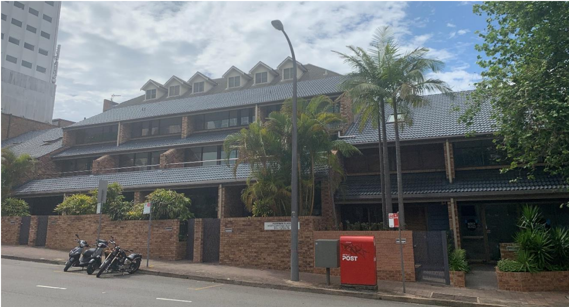
Figure 8 – 263-269 Alfred Street, principal frontage.
