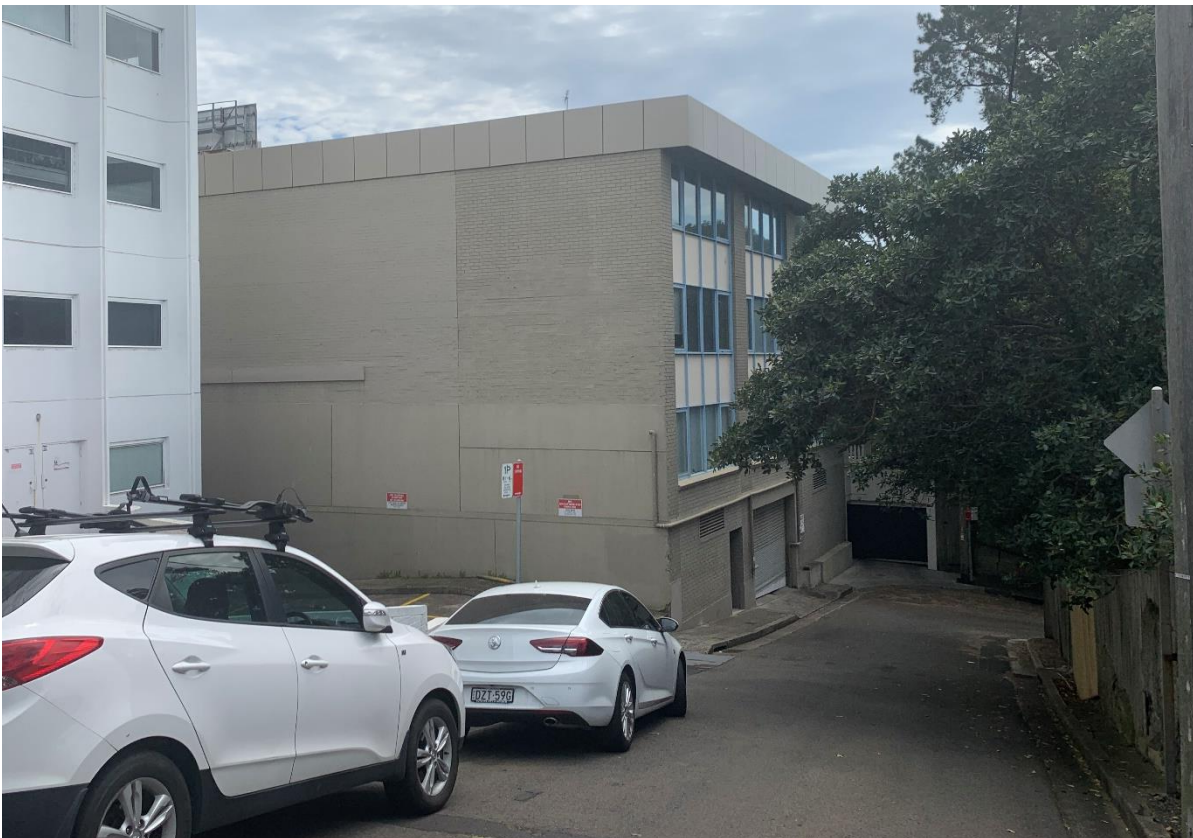
Figure 14 – 283 Alfred Street, rear frontage at Little Alfred Street.
