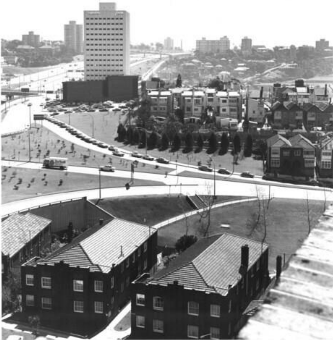
Figure 34 – Warringah Expressway viewed from Greenway Flats, 1975. 'Bayer Building' is indicated. Source: North Sydney File 7619.8.75;68 via Stanton Library, with Urbis overlay
