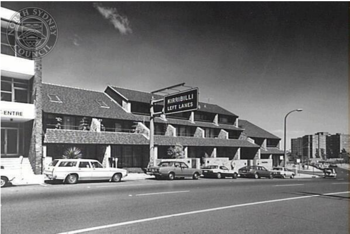
Figure 35 – Primary frontage Portman Place, 263-269 Alfred Street, North Sydney, c1982. Image by Max Dupain. Source: Stanton Library
