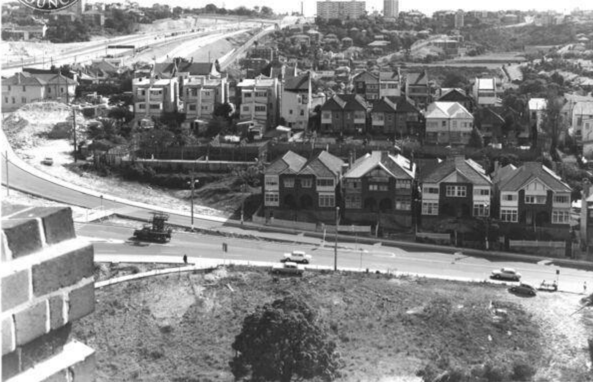
Figure 33 – View of Warringah Expressway, c1960s. Source: Stanton Library
